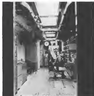
TWO-MAN CREW CONTROLS a flight of Minuteman missiles from a launch control facility of the 141st Strategic Missile Wing at Minuteman AFB, Mont. Firing of a Minuteman flight requires cooperation of two separate launch control centers and the four crew men, who each have to meet and turn keys in five panels. Panels are 10 ft apart to prevent one man from turning two keys in his center.
